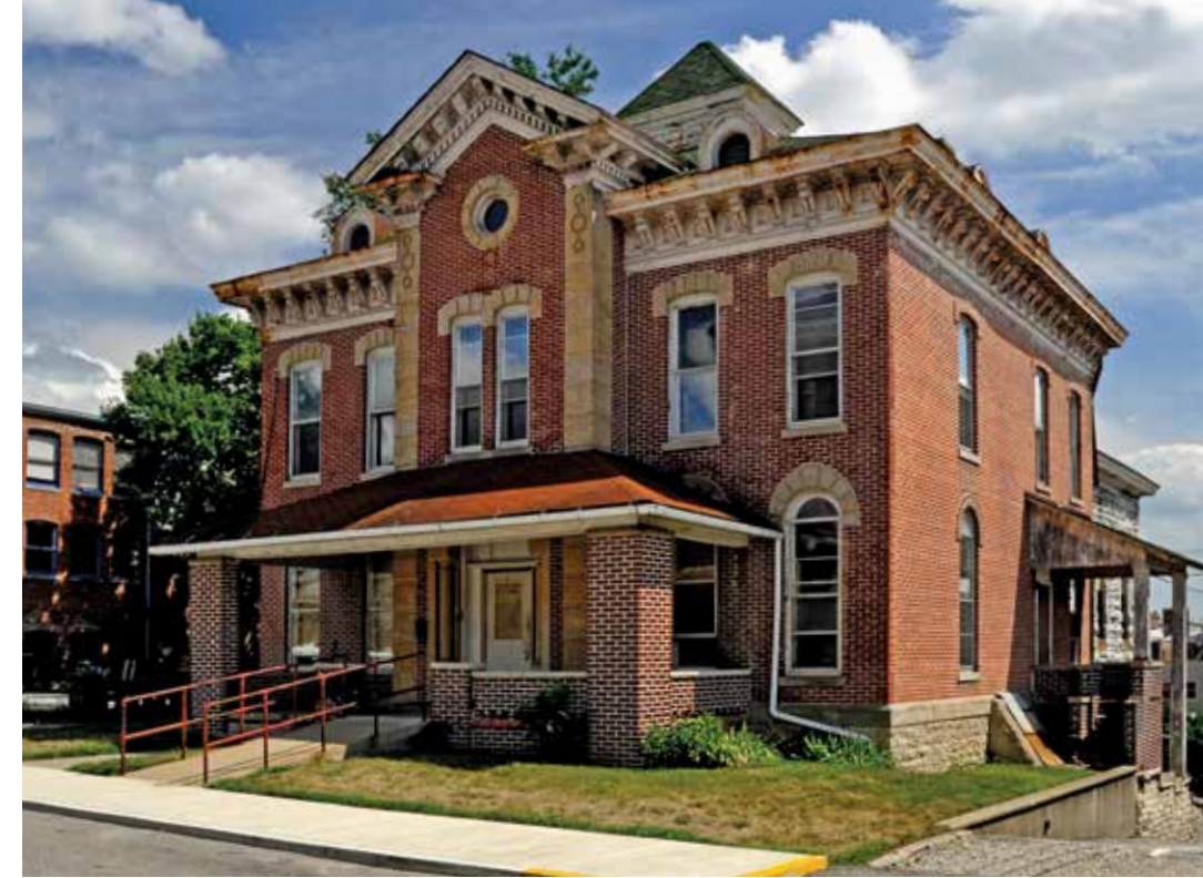
ABOVE: Wabash County Commissioners agreed to give Indiana Landmarks the vacant Wabash Sheriff's House and Jail, another former 10 Most entry, when it was threatened with demolition. We'll make immediate repairs and find a use that ensures the building's future. PHOTO BY LEE LEWELLEN
