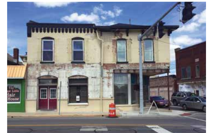
BELOW: In 2011, downtown Greenwood landed on our 10 Most Endangered list when the mayor's renewal plan would have demolished most of the historic buildings. The mayor lost the next election and last year, facelifts were underway on 22 of 33 historic facades. PHOTO BY RAINA REGAN
