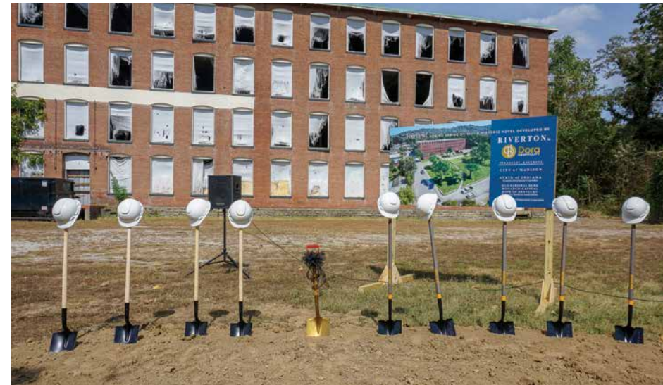
In 2019, Riverton, LLC, the City of Madison, and Indiana Economic Development Corporation kicked off a $21 million project to transform the long-vacant Eagle Cotton Mill, a former entry on our 10 Most Endangered list, into a boutique hotel and conference center. PHOTO BY AUSTIN SCHELL
