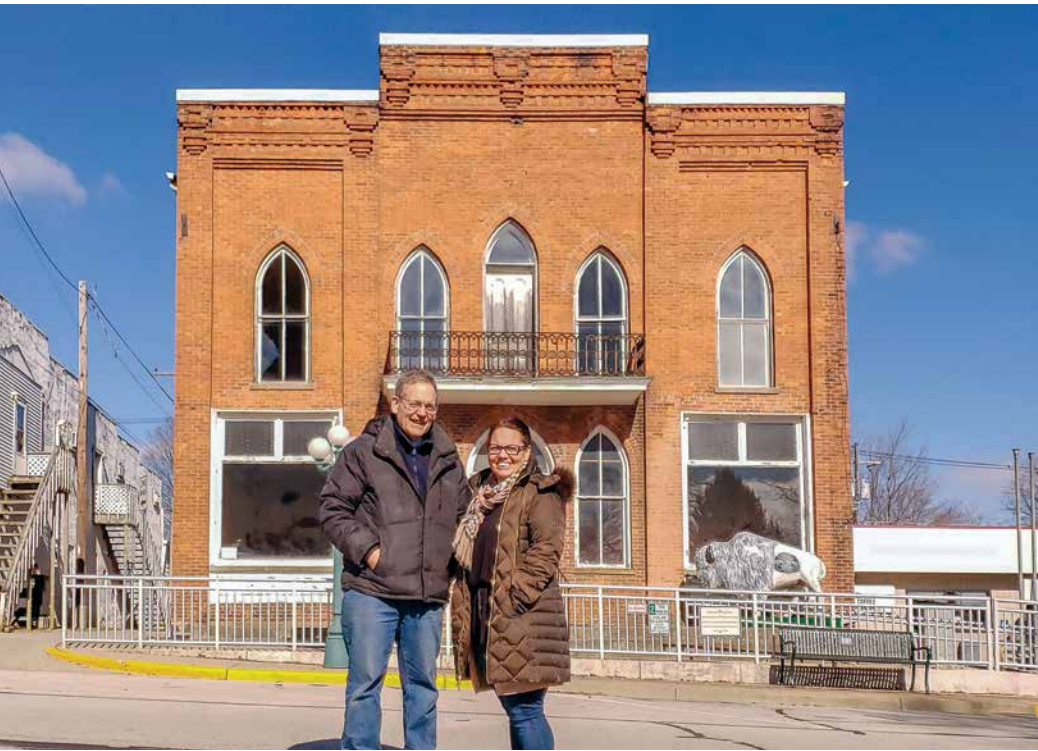
Lawyers Everett and Helen Newman spotted Albion's 1879 Opera House for sale on Indiana Landmarks' website in 2018 and made us an offer, opening their new offices in the lower level. The sale capped a decade of advocacy by local preservation leaders to save the building. PHOTO BY TODD ZEIGER
