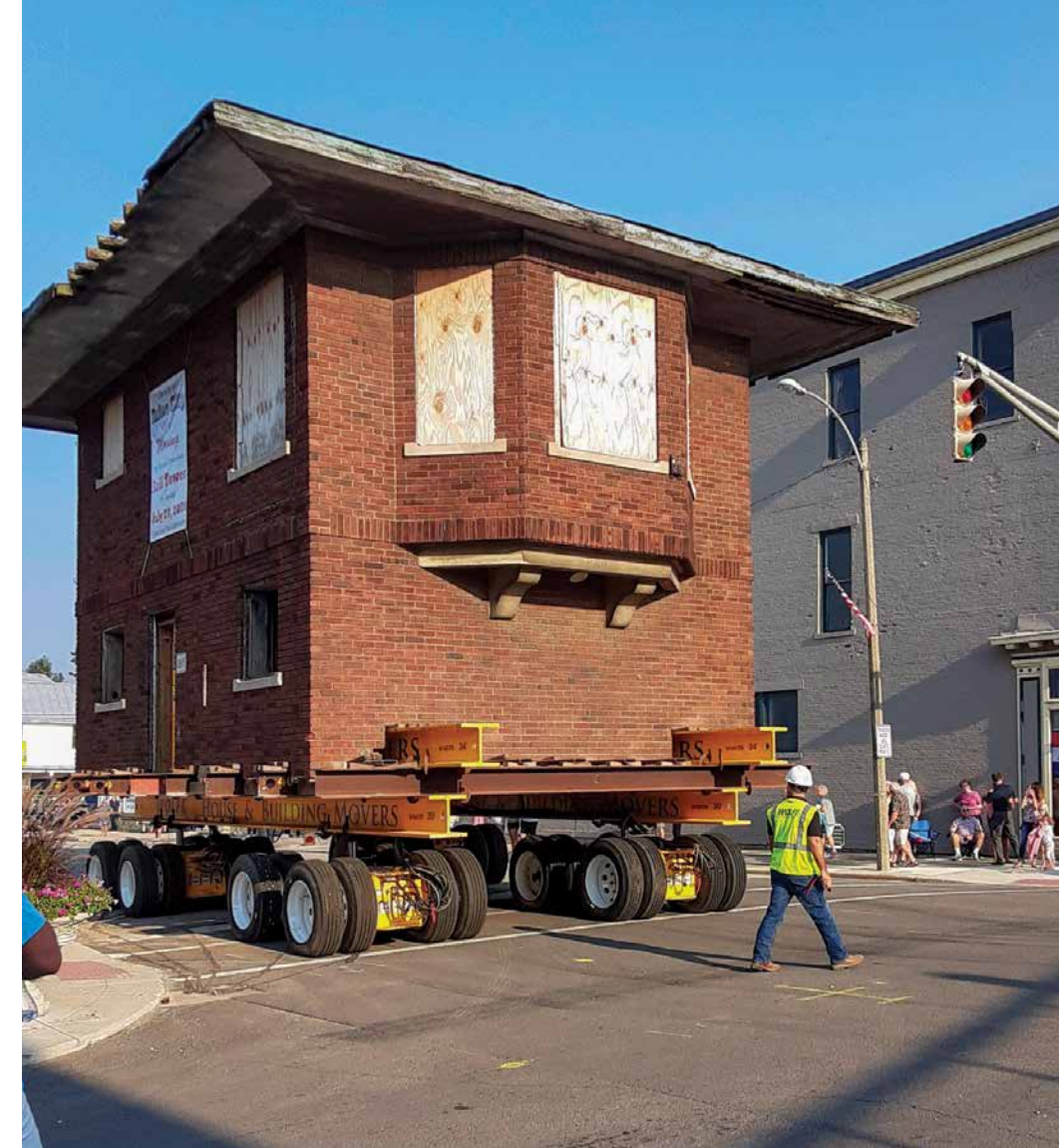
When demolition threatened Union City's 1929 rail tower, Indiana Landmarks' affiliate the Preservation Society of Union City joined community leaders in rallying to save the structure, raising money to move the two-story brick building to a city park, where it will house visitors' information, restrooms, and railroad artifacts. PHOTO BY TED LEAHEY
